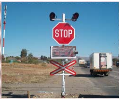
Regulatory signs: Stop Sign (R1) and Flashing lights combination at a level crossing.
