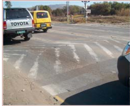
Speed Humps at a level crossing forcing motorists to reduce speed and stop at a level crossing.
