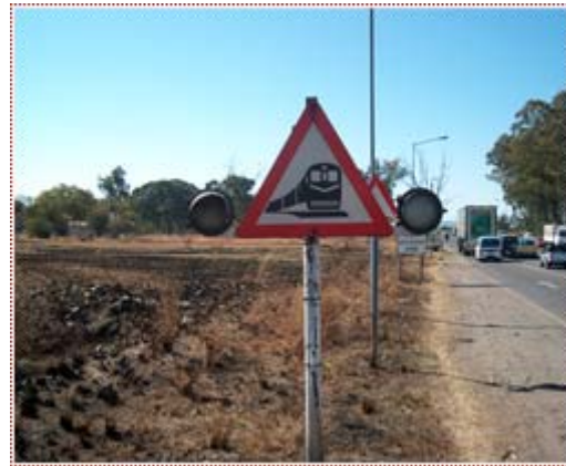
Advance warning sign W318 with flashing lights.
